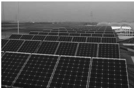
Fig. 2. Photovoltaic generator (45kW peak) on the roof of GE Global Research Europe in Munich.
