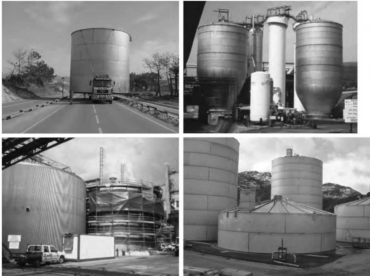
Fig. 5. Storage tanks of duplex stainless steels, SAF 2507 upper left, 2205 upper right, 2304 bottom left and LDX 2101 bottom right.
