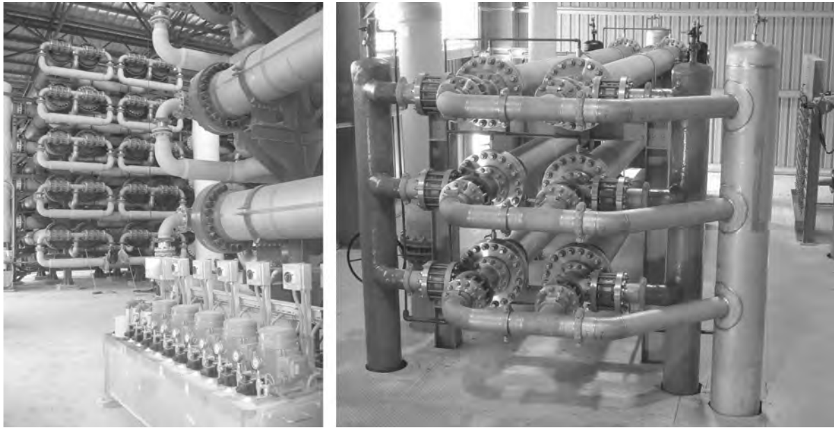
Fig. 2. Energy recovery systems (DWEER) made of SAF 2507 for Ashkelon (left) and Singapore SWRO plants (Courtesy of VID and DWEER respectively).
