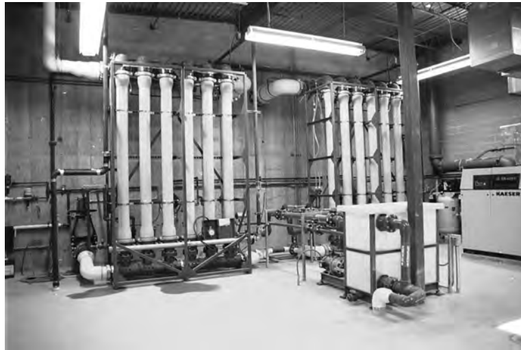
Fig. 3. Full scale NORIT AirLift MBR system.
