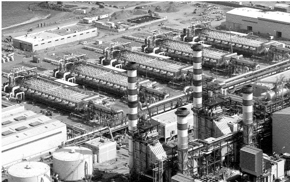
FIG. 20.23 Aerial view of the Fujairah MSF desalination plant.
