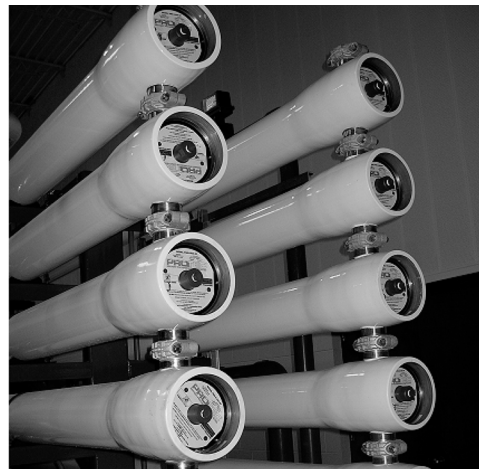
FIG. 5.4 Array of “multiport” pressure vessels (courtesy of Protec Pressure Vessels).
