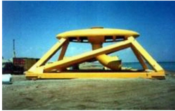
Figure 9 – A submerged type of intake used to supply seawater feed to a desalination plant in Cyprus
