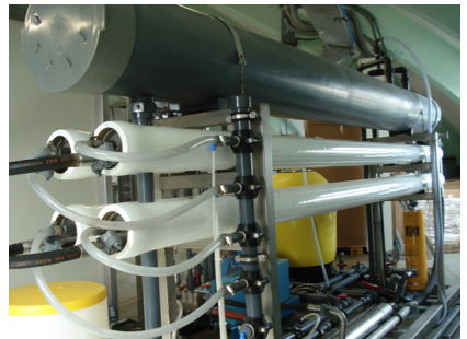
30 mcd solar PV powered RO plant
