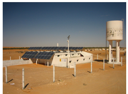
Autonomous solar PV-RO system installed in Tunisia
